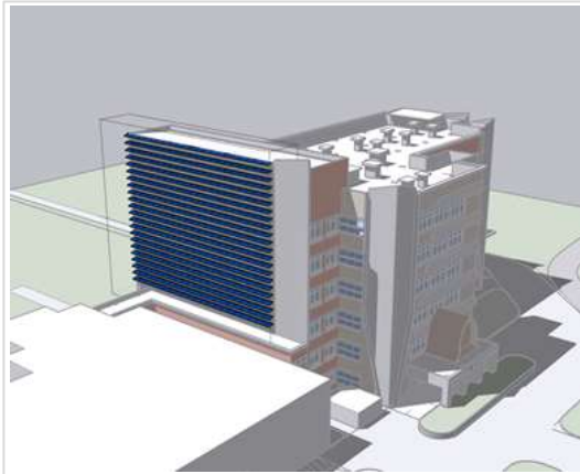
Figure 14. PV simulation on West facade 1 m
