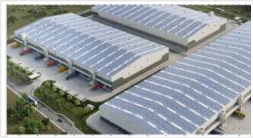
Figure 9. Application of solar panels on rooftops of conserved buildings as utilization of renewable energy
