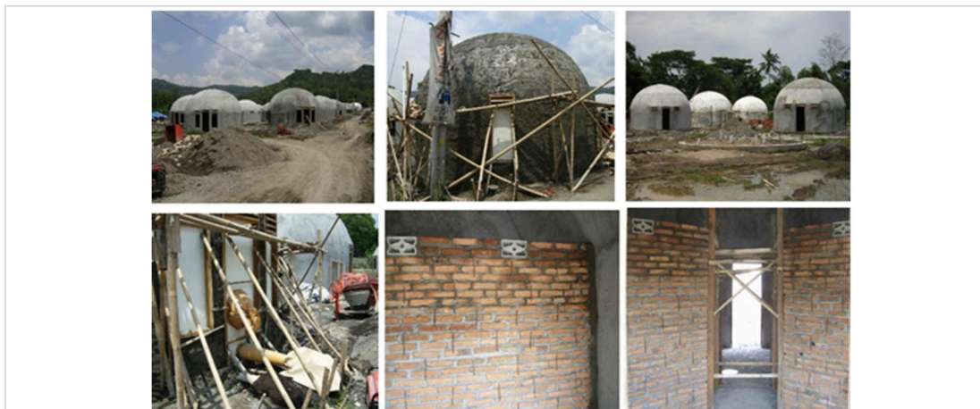
Figure 2. Implementation of the dome house construction process, Nglepen hamlet
