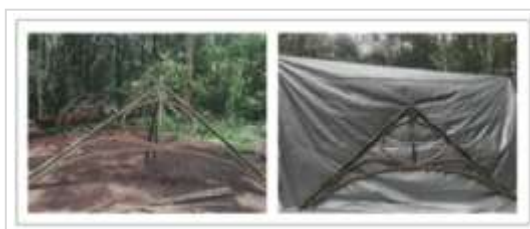
Figure 9. Final truss assembly in bamboo land at 1:1 scale
