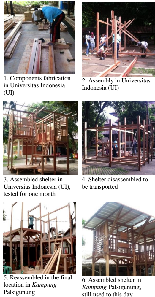
Figure 1. Design and construction process of 'popsyandu' shelter
