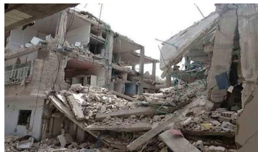
Figure 2. Two-storey building collapses in Gbagada, Lagos Source: (David 2020)
