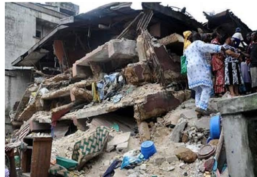
Figure 6. Poor standard of materials Source: (Usman, Akoni, and Olowoapejo 2011)
