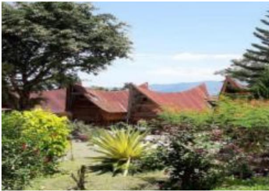
Figure 15. Wood and zinc as the cover material of house buildings Source: (Tobing, Sakti, and Hanny 2020)
