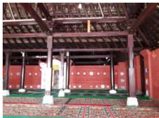
Figure 15. The interior columns' structural and construction system on the Merah Panjunan Mosque building adopts soko guru from Javanese architecture
